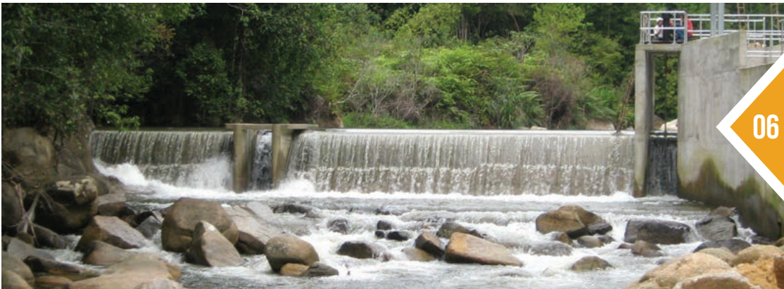
This photo shows the weir structure for the same small hydro facility
